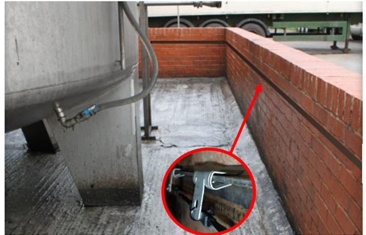
Patol's Linear Heat Detection Cable (LHDC) can be used on the outside of buildings and on the inside of Bund walls to detect excess temperature associated with Fire conditions.
