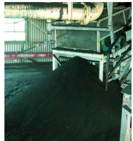
Coal accumulation at a conveyor tail
