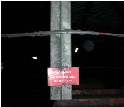
LHD & Catenary Wire Support Courtesy : Patol Limited.
