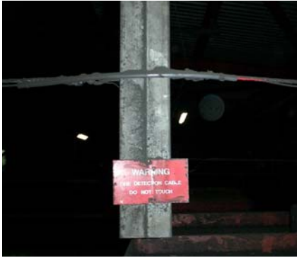
LHD & Catenary Wire Support Courtesy : Patol Limited.
